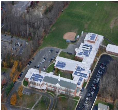
Newtown Middle School solar project completed in 5/1/13 Size of System: 180,000 Watts
