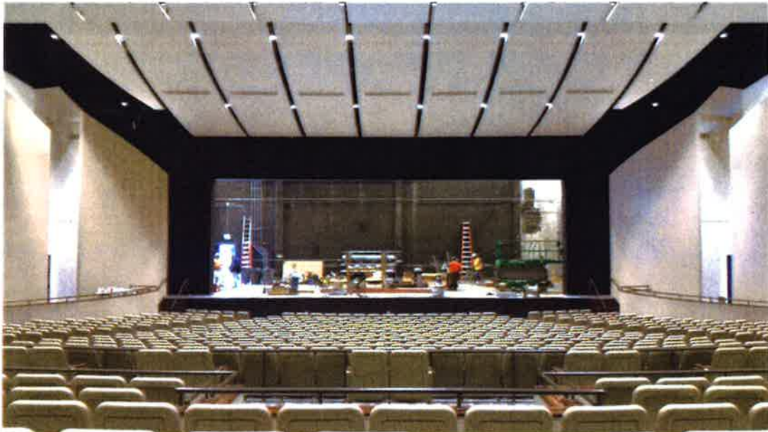
View of House and Stage from Control Booth (9/8/2017)
