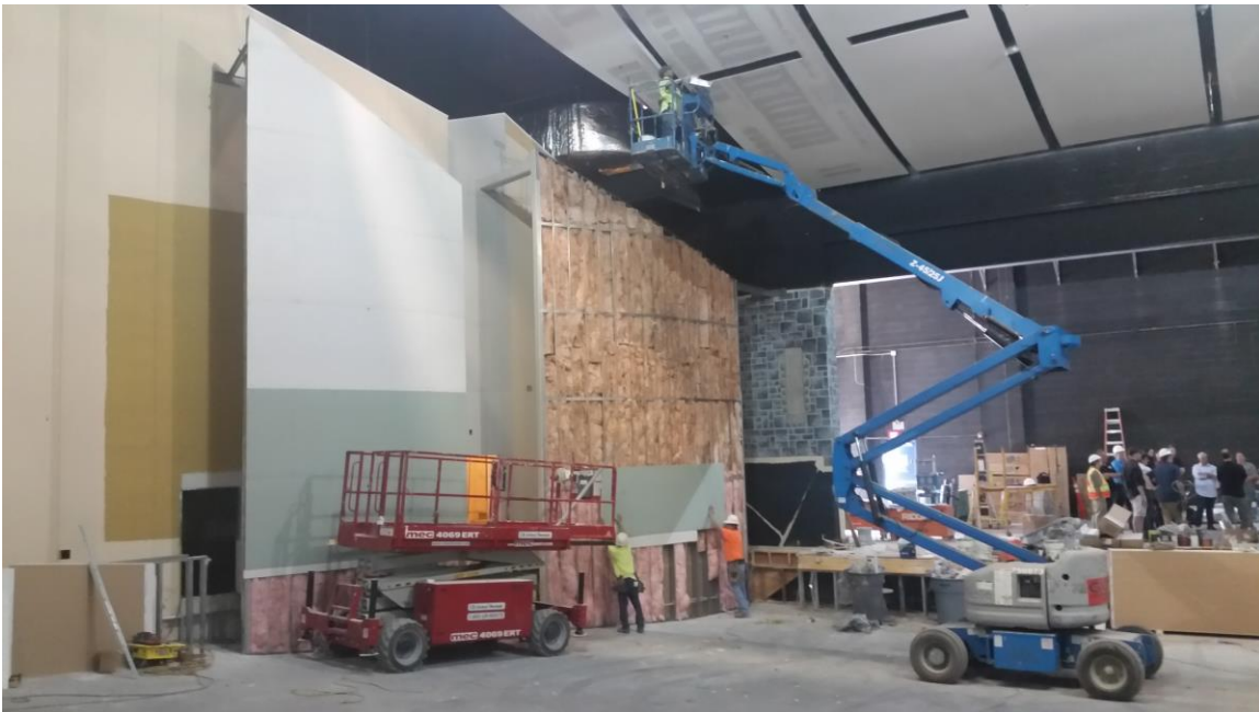
View of Box Seating Walls from Elevated Seating (7/6/2017)
