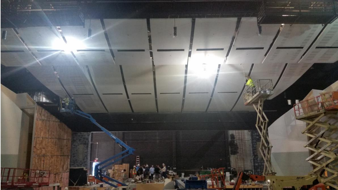
View of Stage and Ceiling Clouds from Rear of Theater (7/6/2017)
