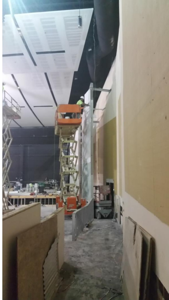
Side Aisle Ramps Behind Box Seating (7/6/2017)
