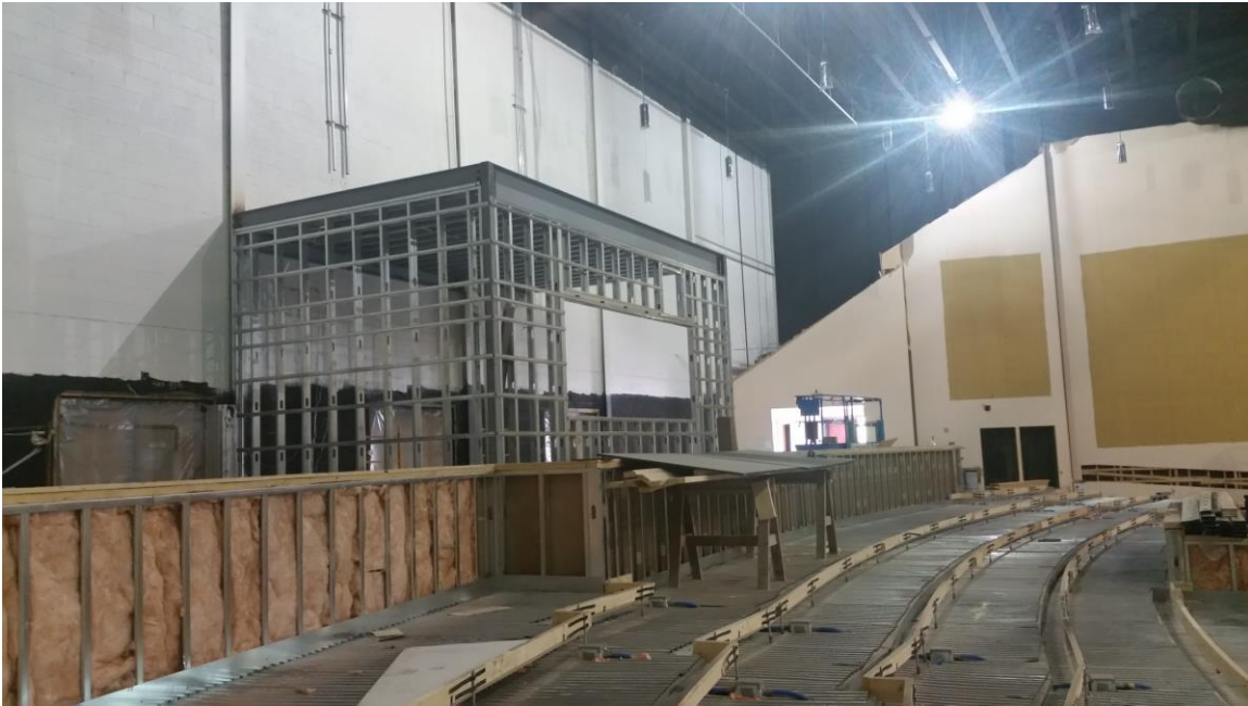
Control Booth & Raised Seating Platform Framing (from rear side aisle) (7/6/2017)
