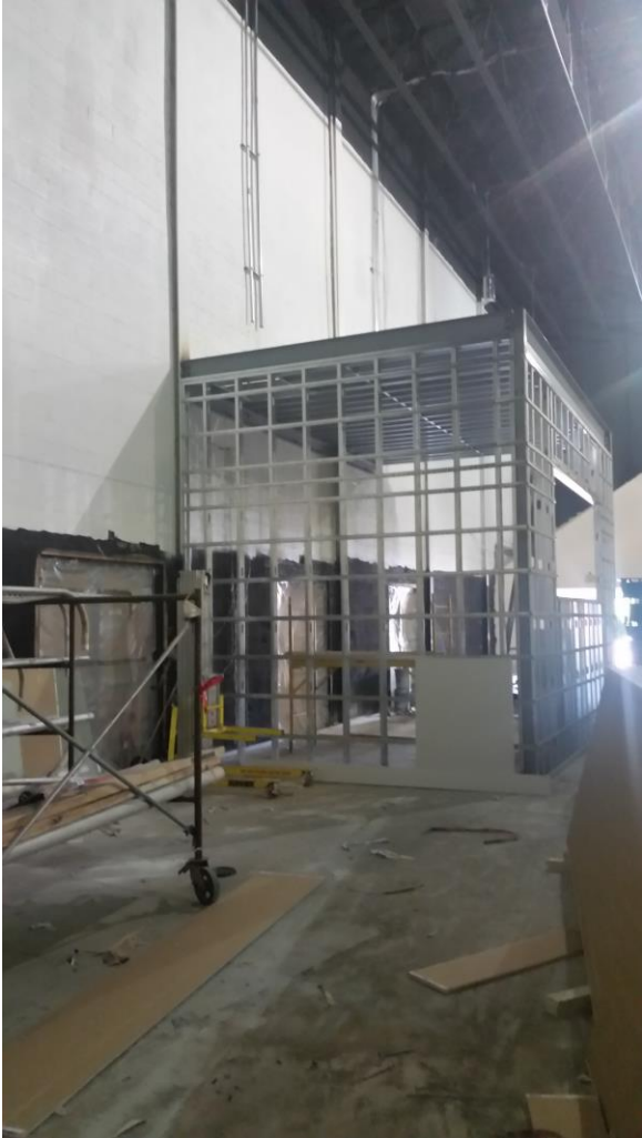
Control Booth Framing (7/6/2017)
