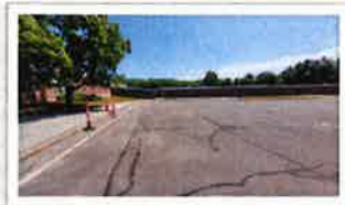
NMS SIDEWALK REPAIR
