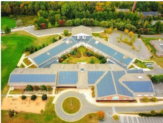
Reed Intermediate solar project completed 8/1/17 Size of system: 635,000 kW
