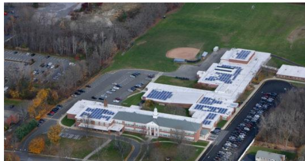
Newtown Middle School solar project completed in 5/1/13 Size of System: 180,000 kW
