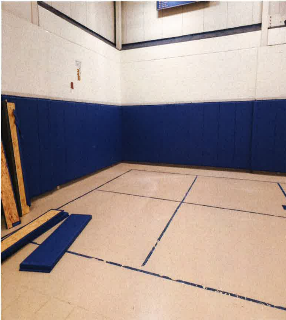
Newtown High School – New wall pads in auxiliary gym
