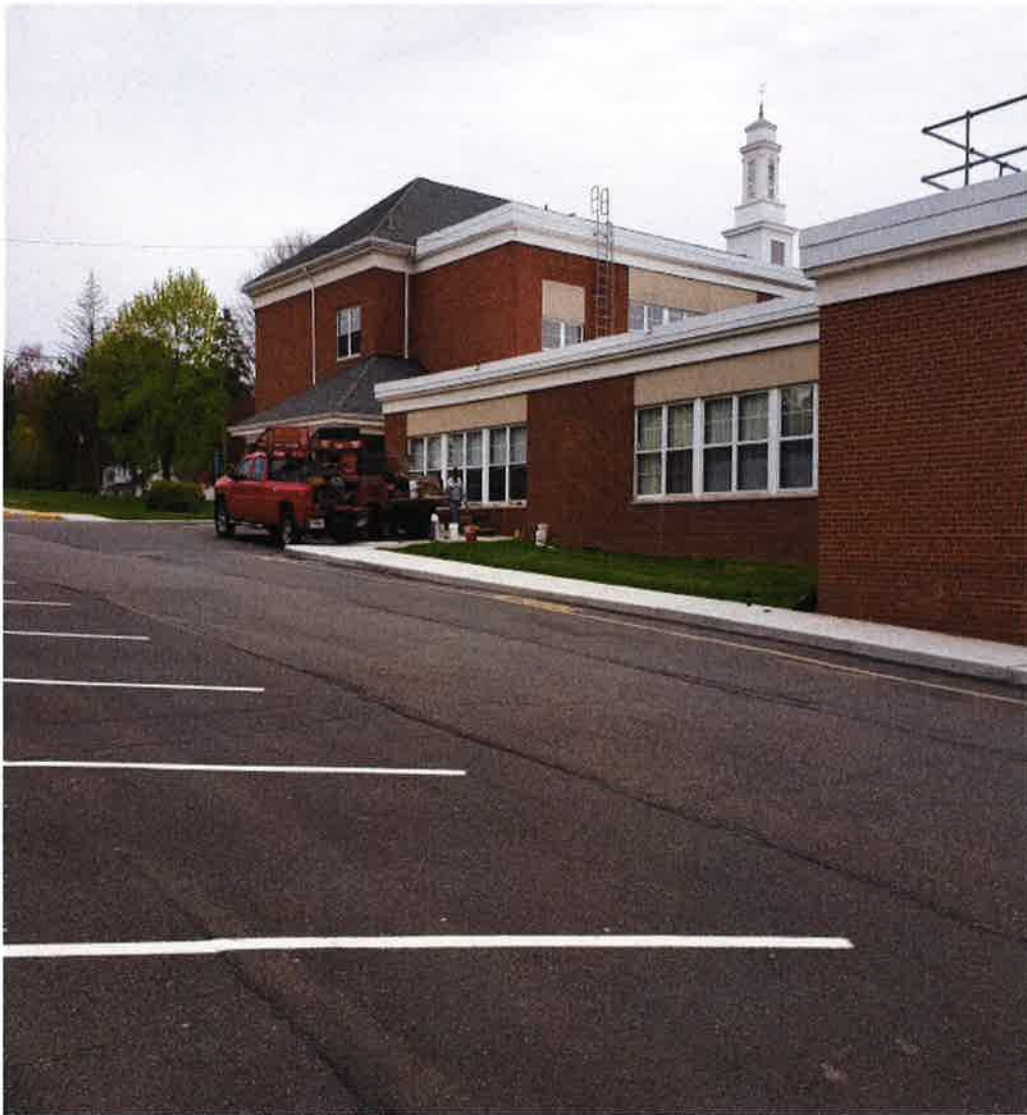
Newtown Middle School – Repointed mortar joints
